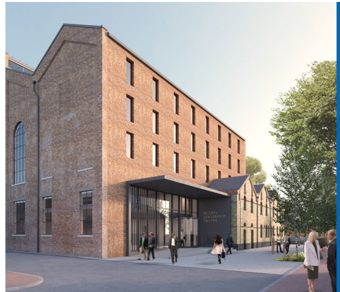
The proposed new entrance to the Global Leadership Centre Image credit: John McAslan + Partners
